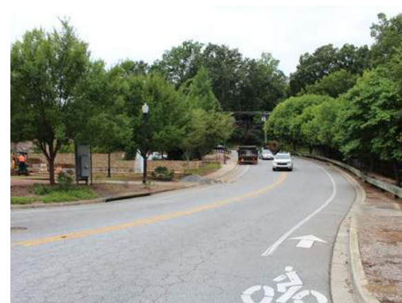
FIGURE 1.D: Bike lane along Edgewood Avenue with limited separation from vehicle traffic
