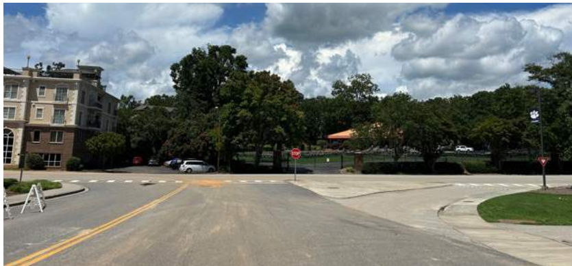
FIGURE 3.D: At SC 93 (Old Greenville Hwy) and Centennial Blvd, drivers turning right use this slip lane with only a yield sign to guide their speed and behavior. Tire marks suggest frequent fast turns through a pedestrian crosswalk, just steps away from student housing and university campus.
