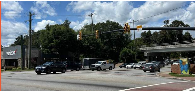
FIGURE 3.C: Intersection of US 123 (Tiger Blvd) and SC 133 (College Ave) is a high-speed, high-conflict intersection due to its combination of fast-moving traffic with frequent turning movements, wide crossing distances, and limited pedestrian protections
