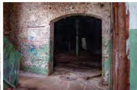
NEWRY MILL INTERIOR ARCHWAY
