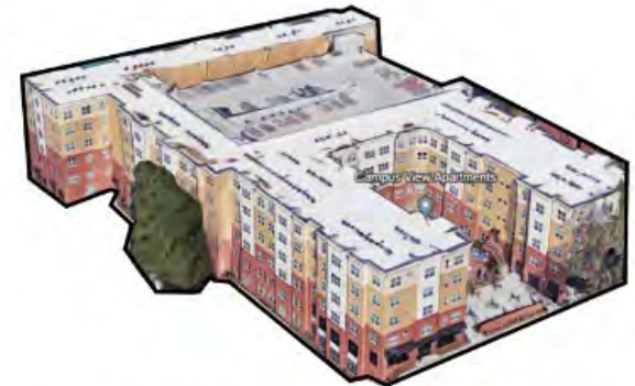
Campus View Apartments: 88'-0", 6 stories
