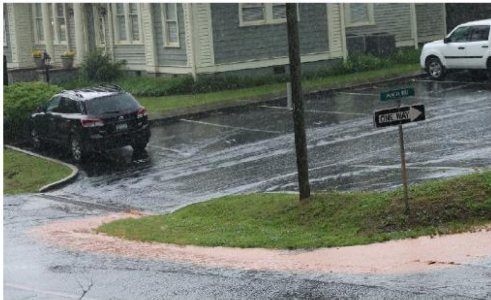
Photo Knox RD at Strode (May 2025 during MODA construction).
