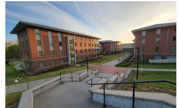
Douthit Hills On-Campus Student Housing, Source: Jonathan Ceci Landscape Architects
