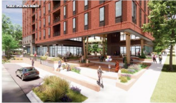
ON SITE CLERMONT © 2014 ARUP CONSULTING INC.
